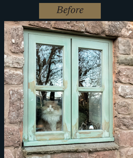
Old, flaking timber windows in need of updating and replacing.
